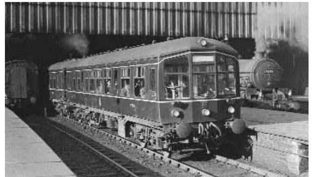
Bradford Exchange: The transition from steam to diesel in the 1960's.
