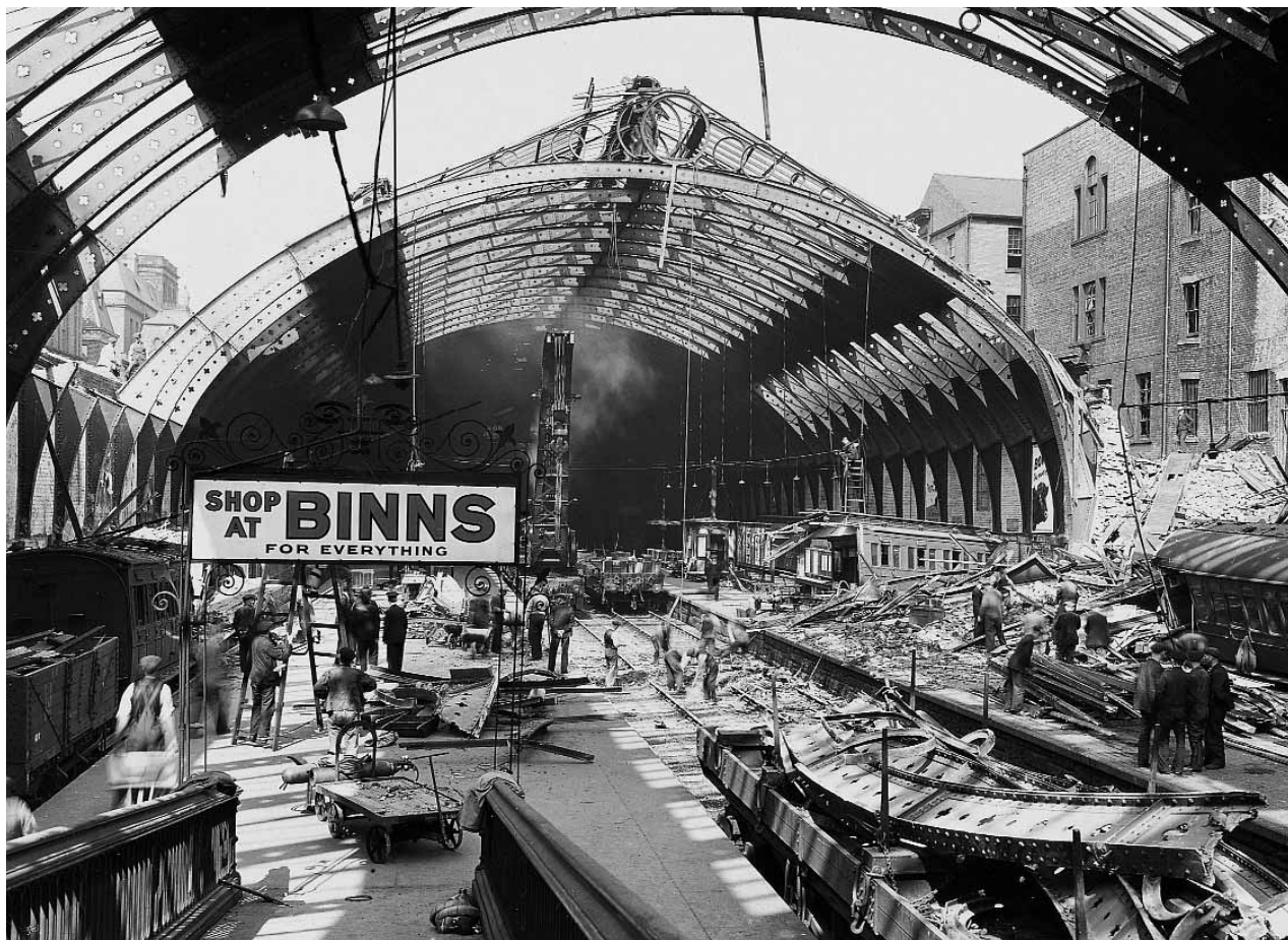
Devastation at Sunderland station during the blitz. Photo courtesy of Backtrack Magazine.
