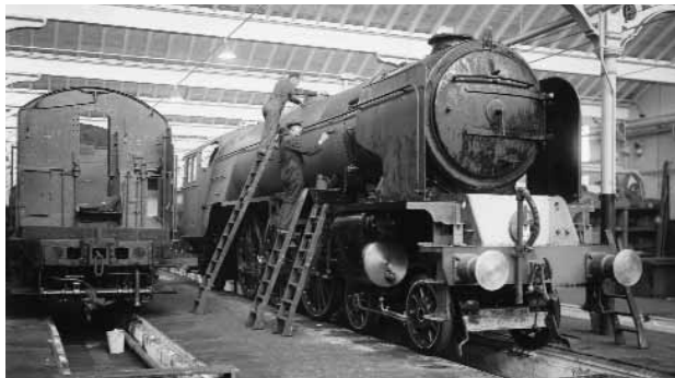
Railway workers painting an A2 class locomotive at Doncaster Works, 28 November 1947.
