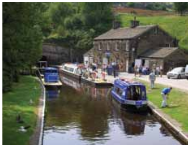
Tunnel End at Marsden © British Waterways
