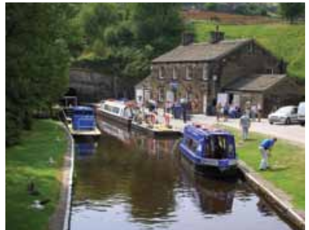
Tunnel End at Marsden © British Waterways
